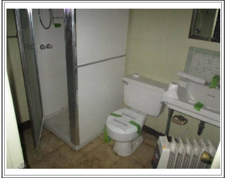
Basement - Full Bathroom
