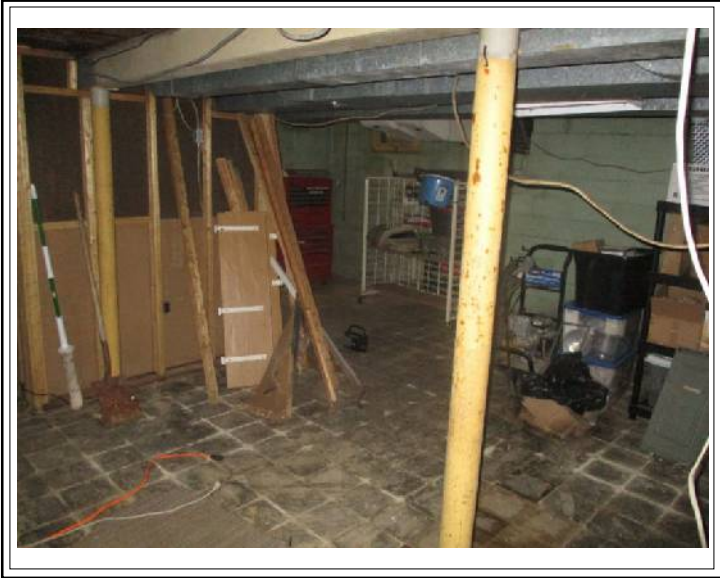
Basement - Unfinished Area - Photo #2
